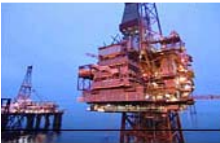
multiphase pumping module, Dunbar, North Sea
