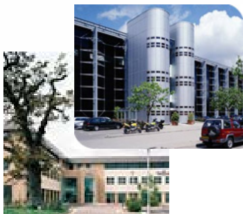
Data & Application Support Centre
